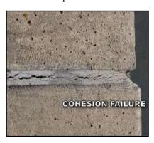
results when the sealant material itself splits or otherwise opens allowing moisture to flow into the building.
